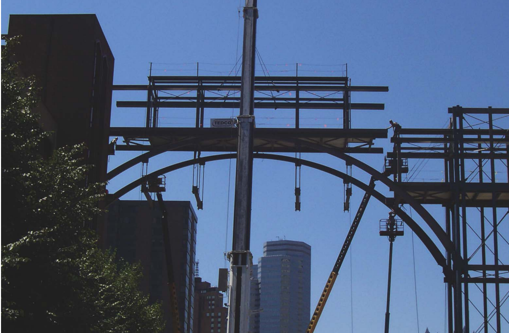
Above: One inch was allowed for tolerances when erecting the prefabricated center span.
