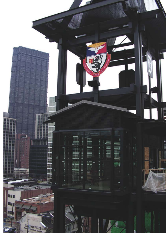
Right: The tower columns support the pedestrian bridge; access to the bridge occurs through the adjacent structures.
