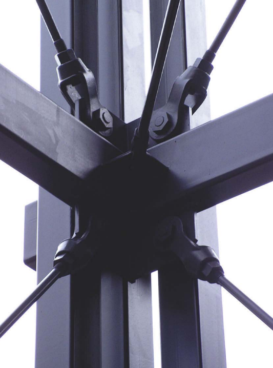
Steel rods and clevises provide visually unobtrusive lateral bracing for the supporting towers.
