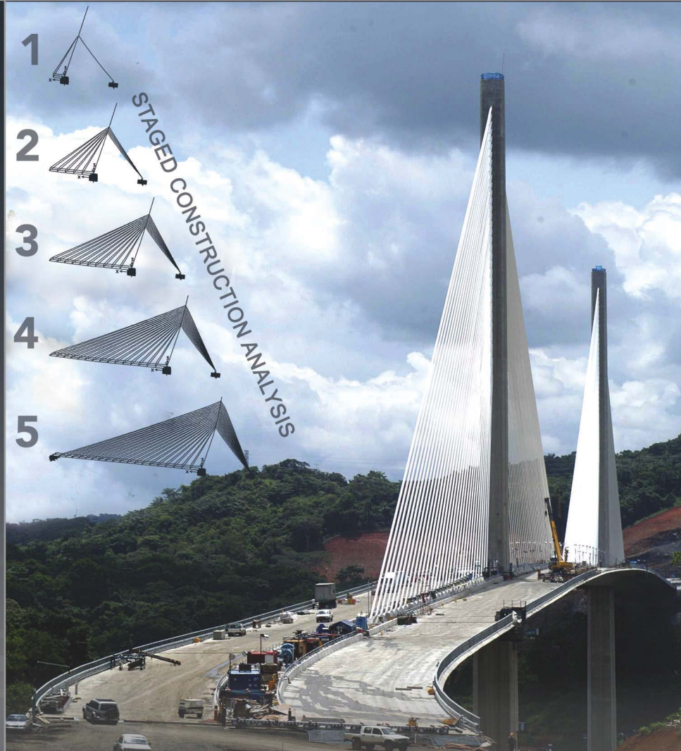
Centenario bridge across Panama Canal the longest concrete cable-stayed bridge. Designed with SAP2000. Courtesy T.Y. Lin International, San Francisco.
