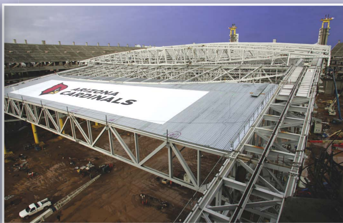
2007 IDEAS 2 National Winner – 400 tons of 12 inch square tubing curved for the retractable, lenticular roof trusses. The University of Phoenix Stadium. Phoenix, AZ.
